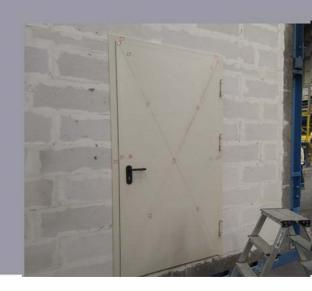
Standard EN 1634-1 Fire Resistance E Class: 120 Min. El Class 30 Min. Width: Max. 1150 mm **Dimension** Height: Max: 2250 mm 1.5 mm DKP or Galvanised Fra me 1 mm DKP or Galvanised Wing Wing Thickness 50 mm Isolation 150 kg/m3 Rockwool Kerafix Intumesan Seal Fire Seal 2 pcs hinges, one of Self-Spring, both are Twisted from 3 Hinge mm Sheet Metal **Desired RAL Color Static Paint** Paint
